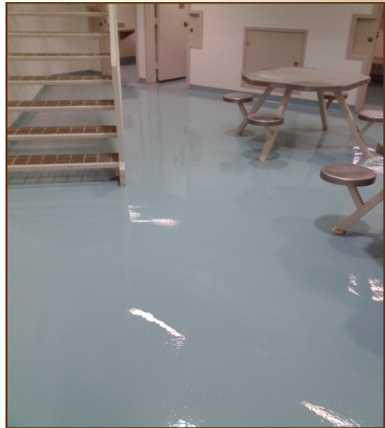
Above and Left: Various phases of the jail's Second Floor abatement process
